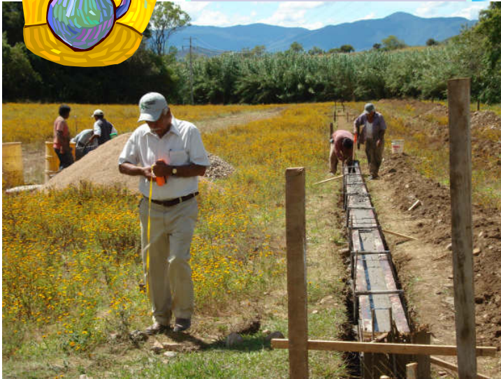
the crew and the infrastructure construction
